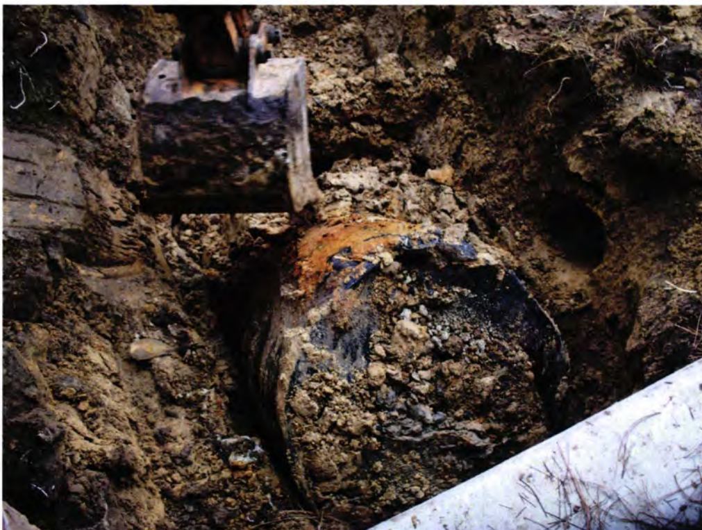
Picture 2: UST 456Elderberry-1 being removed from the excavation.
